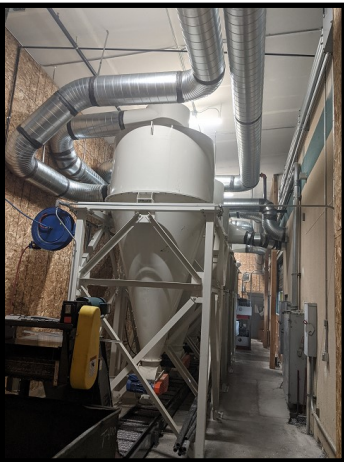
Cyclone Room for Chip Drop-Out
