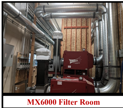
Cyclone Room for Chip Drop-Out
